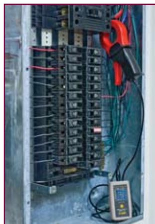
L101 recording branch circuit current.
