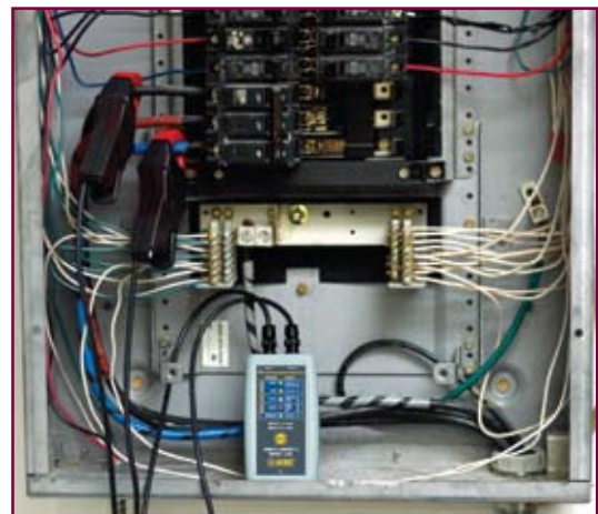
L102 recording two phases of primary feed.
